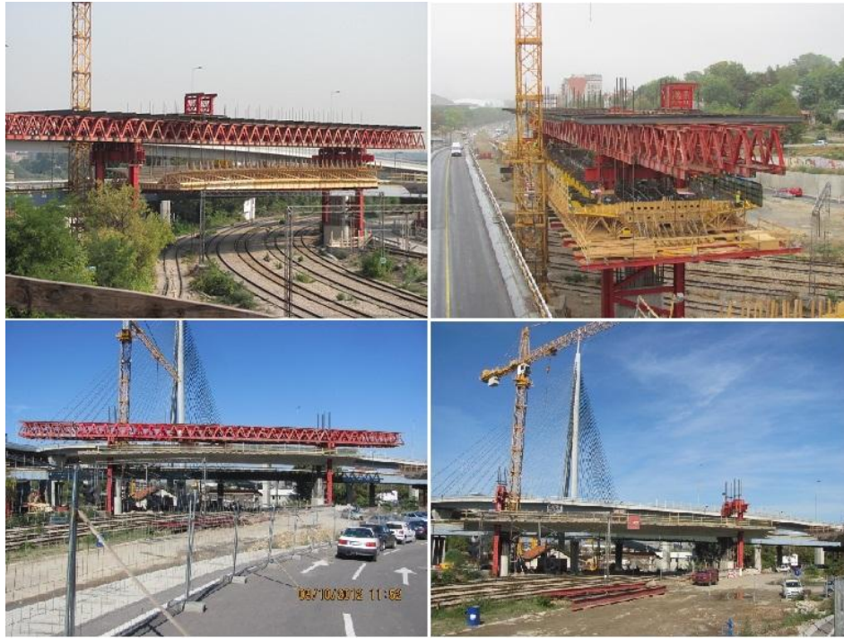
Photos 7-10. NAR – Main construction stages of viaduct in Radnicka street
