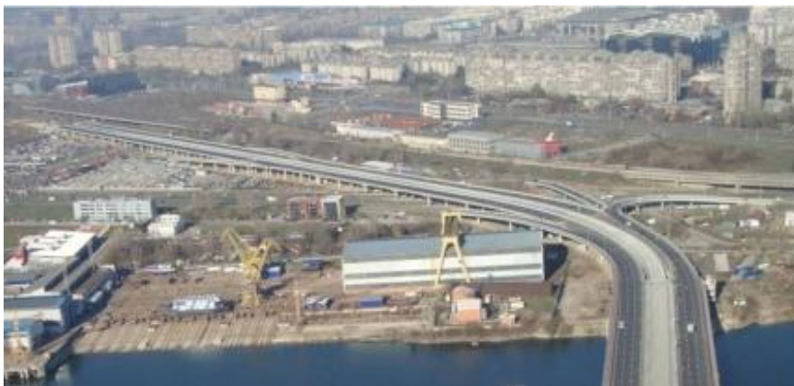
Photo 3. NAR – Viaducts with ramps
