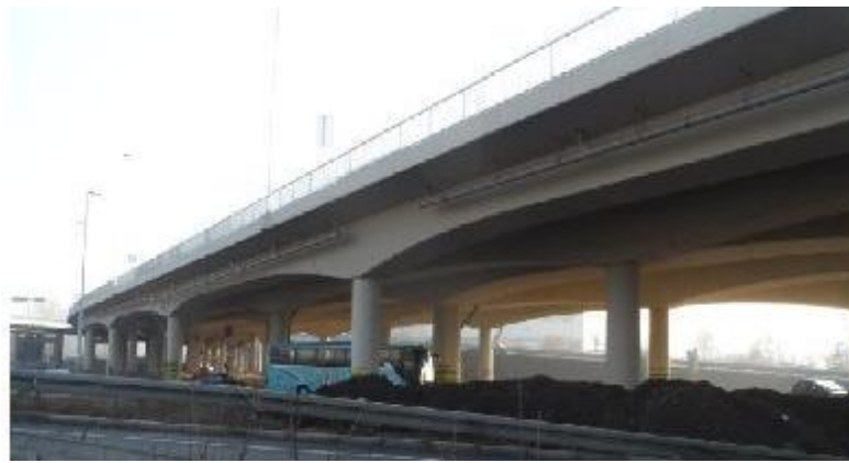
Photo 4. NAR – Viaducts over J. Gagarina street
