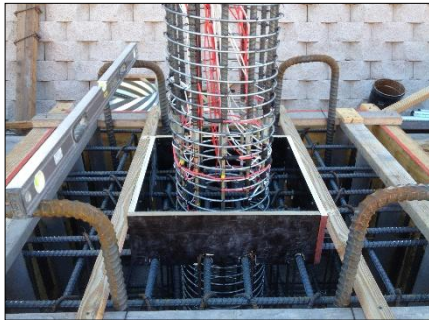
Figure 7. CuAlMn SMA bars in the plastic hinge Figure 8. Completed concrete in the footing and breakout for ECC.
