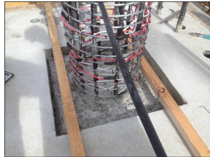
Figure 7. CuAlMn SMA bars in the plastic hinge Figure 8. Completed concrete in the footing and breakout for ECC.
