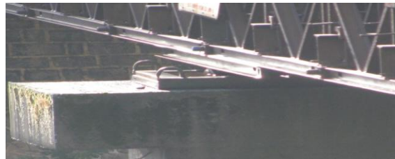
Photo 5. Intermediate support detail
