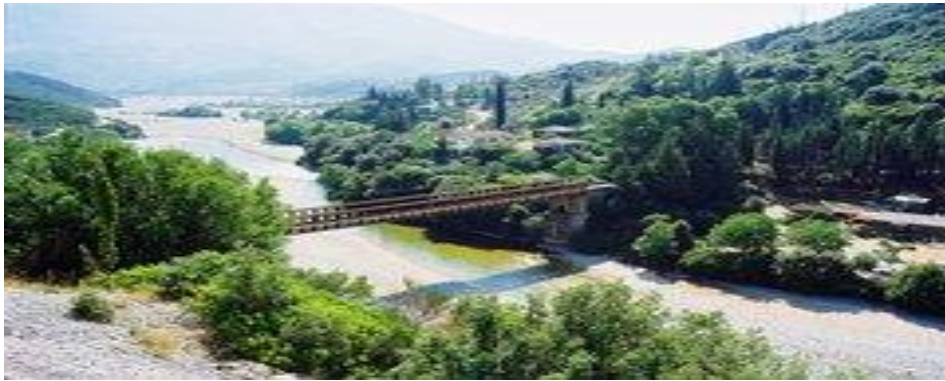
Photo 1. The Bania bridge up to 1986
