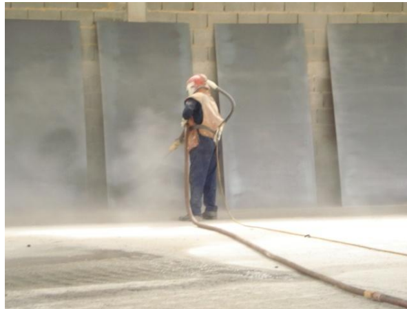
Figure 3. Sand and Soda Blasting
