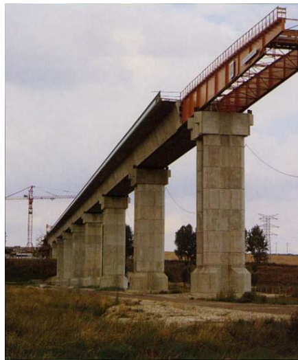
Figure 1. Incremental bridge launching [1]
