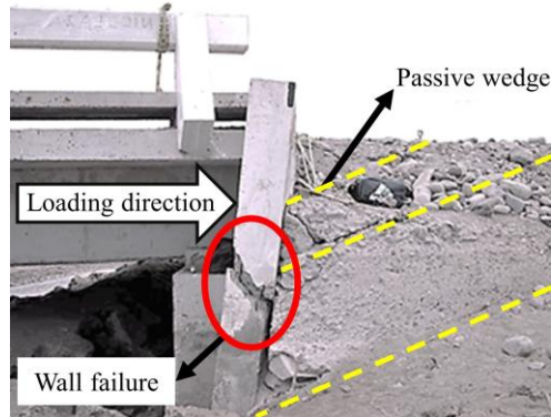
Figure 1. Abutment wall failure under horizontal loading and passive wedges mobilized behind the wall, modified from [3].
