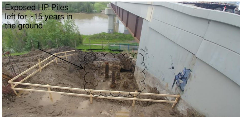
Figure 8. Exposed HP steel piles at abutment (TYP)
