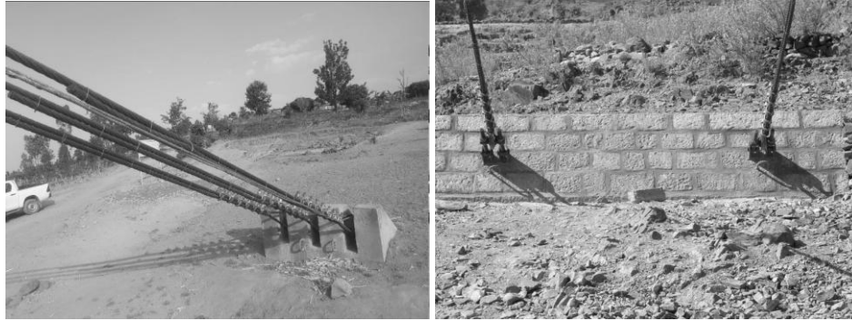
Figure 7. Anchor block, left B2P construction in Rwanda, right Ethiopia practice
