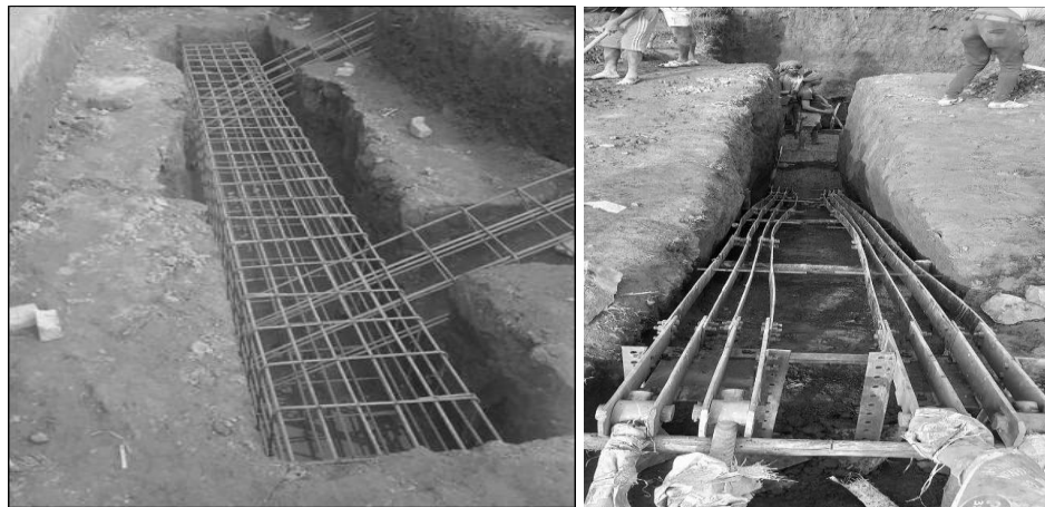
Figure 8. Anchor block transition arm, right B2P construction in Rwanda, left Ethiopia practice
