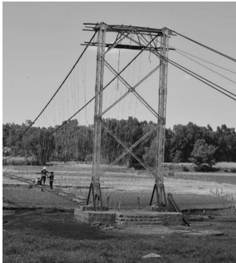
Figure 5. Steel tower, Rwanda style
