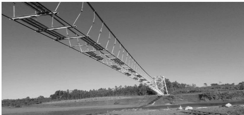
Figure 2. 120m long suspension Bridge under construction in Ethiopia
