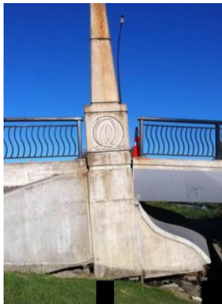
Figure 7. Back-rotation of the south abutment (reprinted from GEER [30]).
