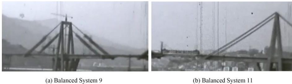
Figure 18. Construction sequence differences between balanced system 9 and 11 (frame from [22])
