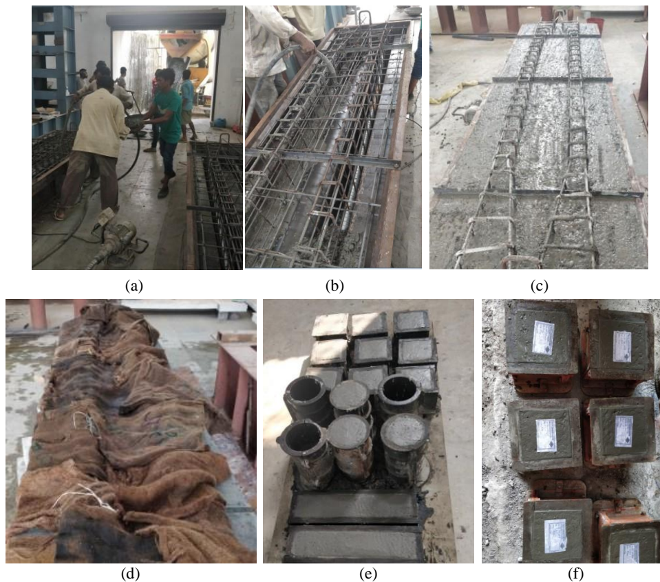
Photo 2. Stages of casting, a) Concreting using ready mix, b) needle vibration, c) Concreting completed, d) Wet sack curing, e) & f) sampling
