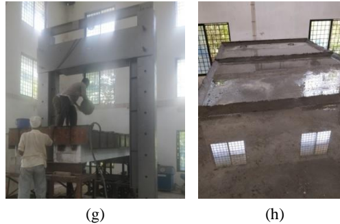
Photo 3. Stages of pre-stressing and casting of integrating slab, g) Concreting of deck slab and h) Curing of deck slab.
