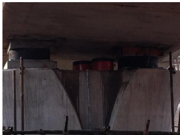
Figure 6. The using LRB in bridges (Photo by Saman Mansouri)
