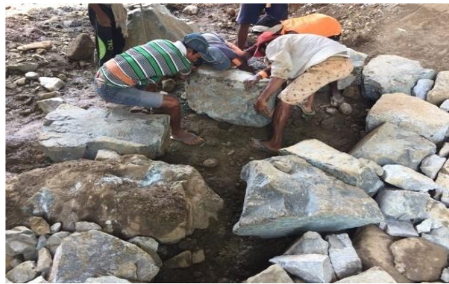
Photo 5. Construction of U.C.R apron
