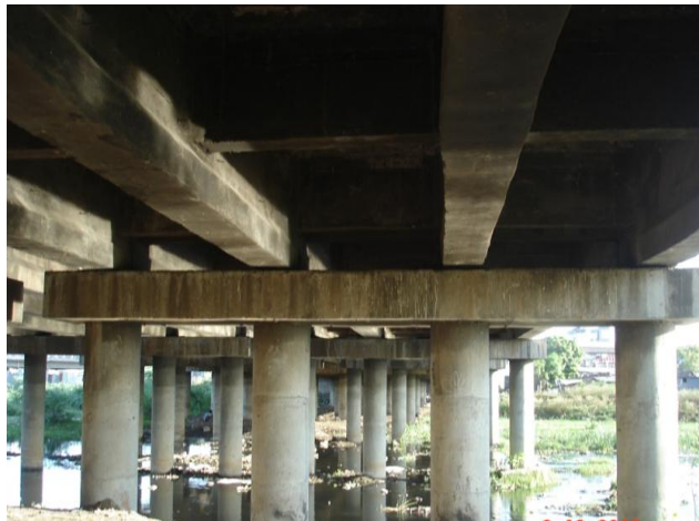
Figure 2. Elevation of the bridge bent
