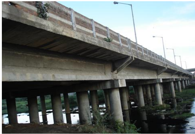
Figure 1. Longitudinal view of the study bridge
