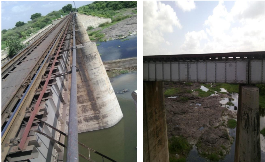
Photo 1. Plate girder bridge on Lalpari River in Rajkot
