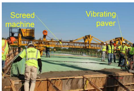
Figure 12. Vibrating paving machine and screed the machine during construction
