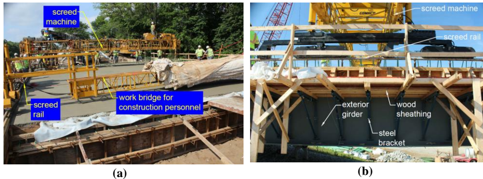
Figure 2. Concrete pouring and finishing work using screed machine
