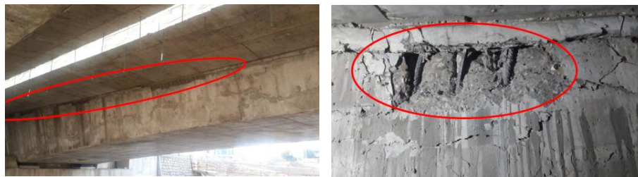
Figure 16. Cracks and concrete scalping at interface (photo courtesy of Mega)
