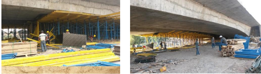
Figure 12. Shore removing and form stripping
