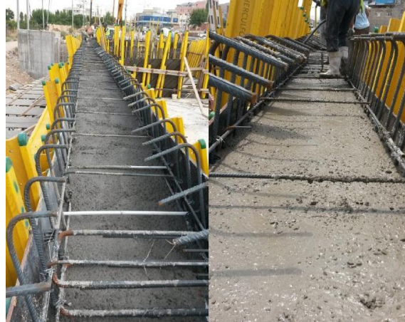
Figure 18. Top surface of the walls left as is without roughening
