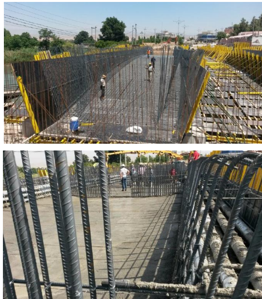
Figure 9. Installation of conventional reinforcement and PT ducts
