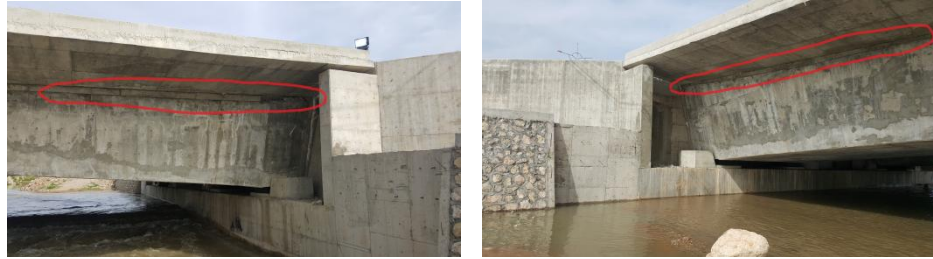
Figure 15. Cracks at interface from both ends
