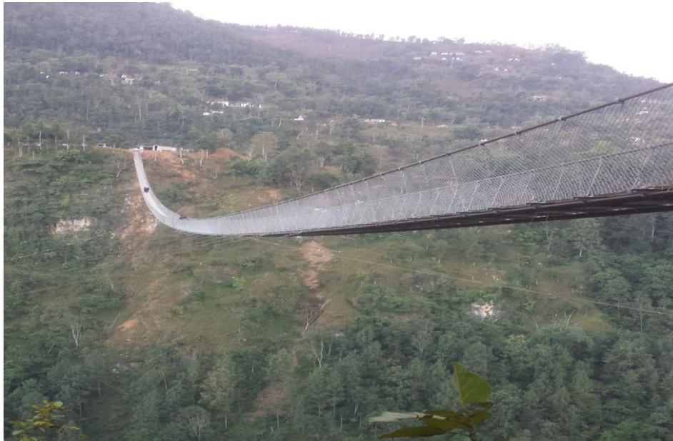
Nepal's longest suspended bridge in Parbat district of Western Nepal
