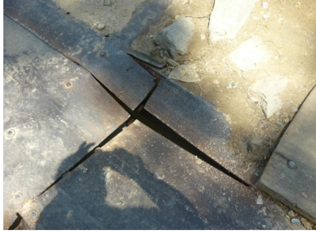
Figure 4. Condition of Decking System
