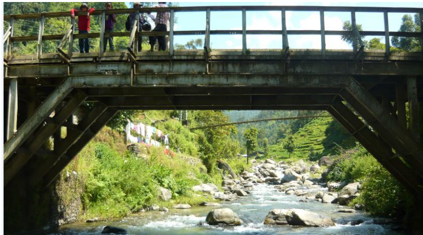
Figure 3. Structure of the Bokse River Bridge
