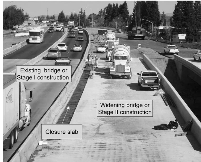
Figure 1. Lane addition by widening or stage construction
