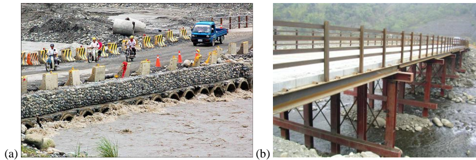
Figure 2. The most commonly used temporary rescue bridges in Taiwan, (a) temporary roadways made from concrete pipes, and (b) temporary steel bridges
