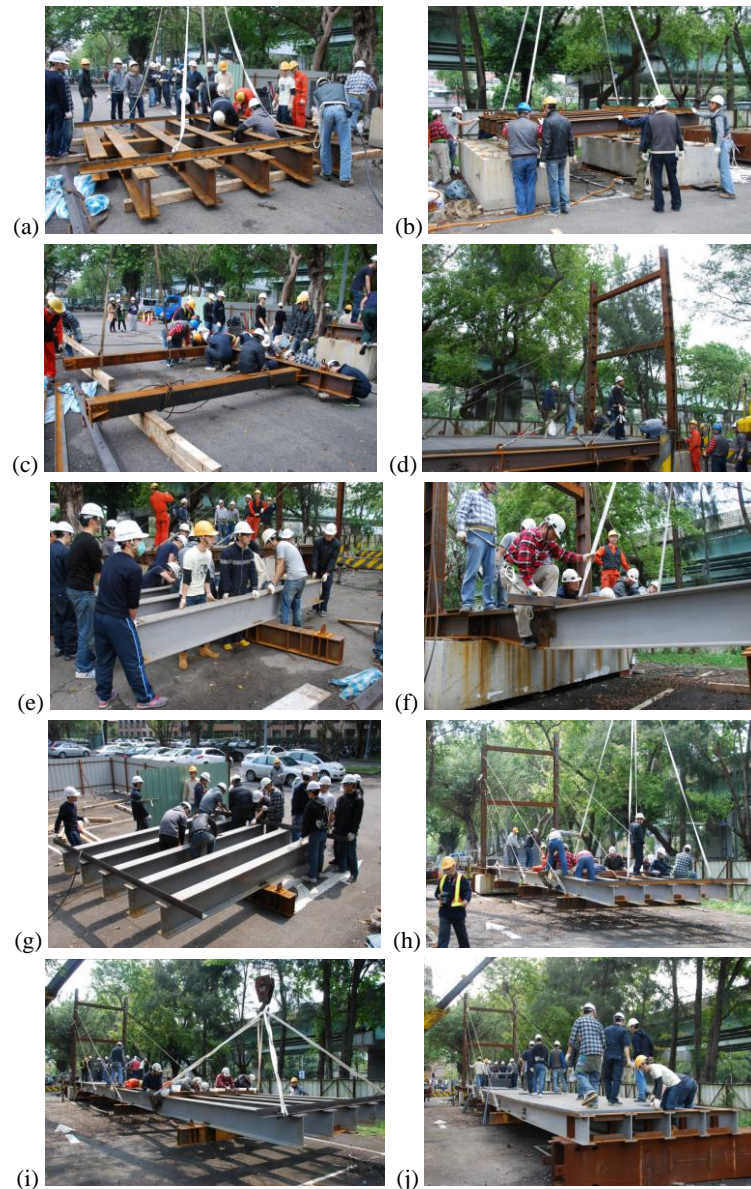
Figure 12. Construction sequence of the 20-m span temporary rescue composite bridge: (a) assembly of seven parallel steel girders; (b) connection of the weight-balance structural module; (c) assembly of the double-H-shaped pillar; (d) connection of the bridge-tower structural module; (e) assembly of the first segment of GFRP girders; (f) connection of the crossing structural module; (g) assembly of the second segment of GFRP girders; (h) and (i) connection of the crossing structural module; and (j) completion of the composite bridge construction
