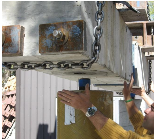
Figure 5. Cap beam installation
